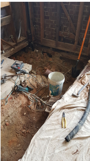
Flooring opened to inspect and repair termite-damaged areas.
