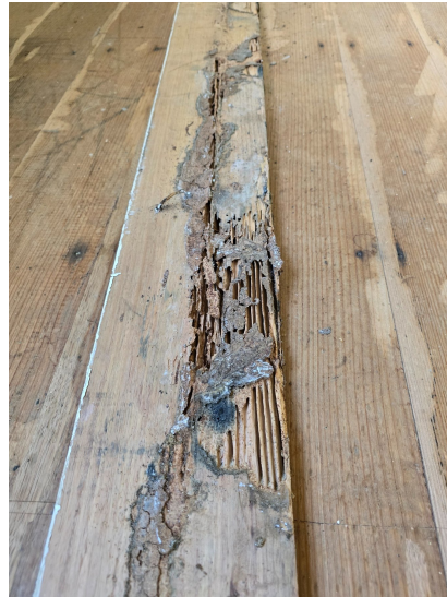
Subfloor/foam repair during rectification.
