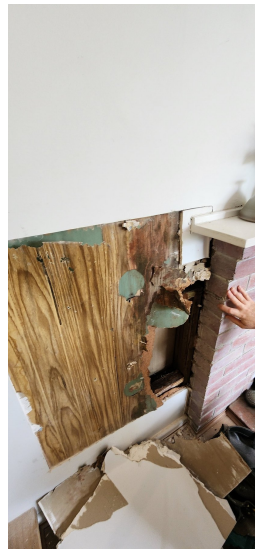
Framing repair around exposed services and old wall construction.
